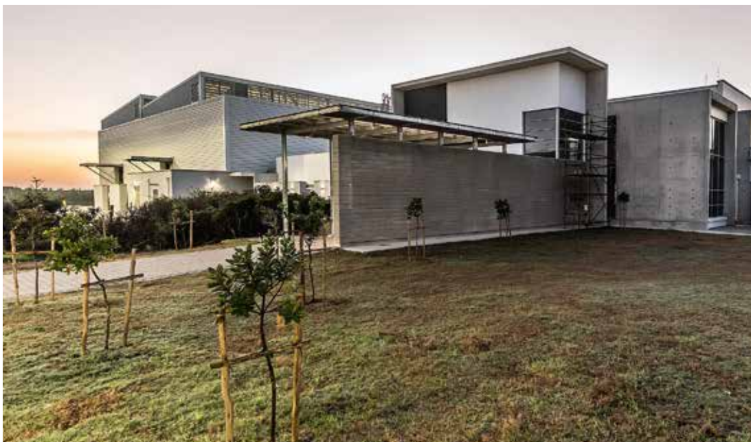
The walkways around the courtyard edge include plenty of glass and natural ventilation. The tranquil gurgle of the courtyard water feature dampens noise from the N2 highway and the testing laboratories.
